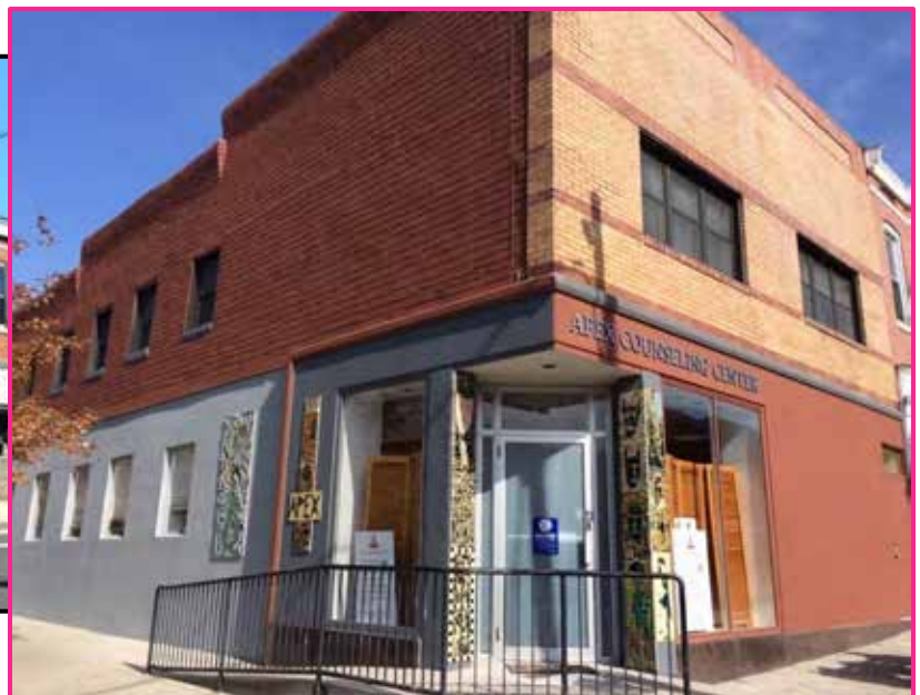
After at 3200 Eastern Avenue. Work included brick cleaning & repointing, repairs to cracks in the stucco siding, and painting.
